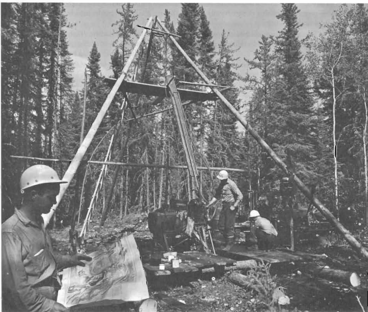
PLATE III Diamond drilling. Drills probe deep beneath the surface to locate possible mineral deposits suspected as a result of geological studies, airborne geophysical surveys, and ground geophysical surveys.
