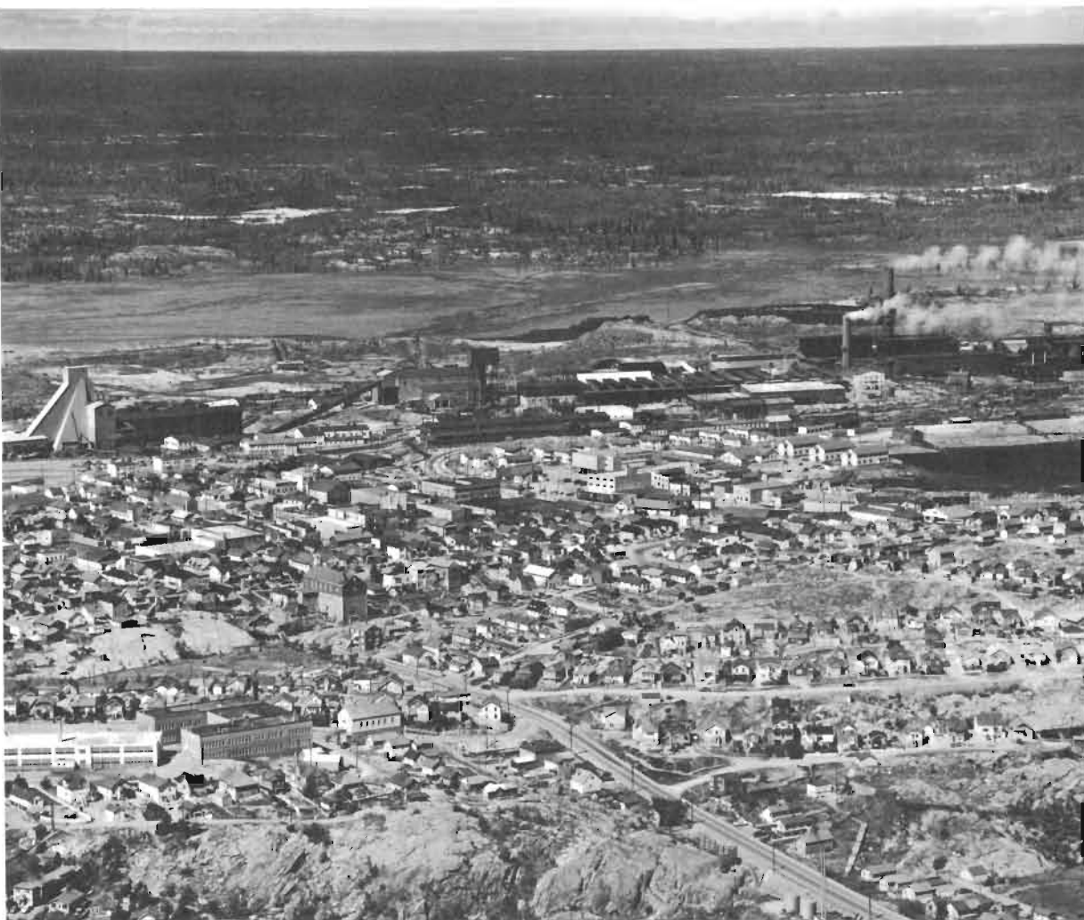
PLATE VIII Flin Flon, looking west. Behind the mine area is Flin Flon Lake, now filled with tailings from the mill.
